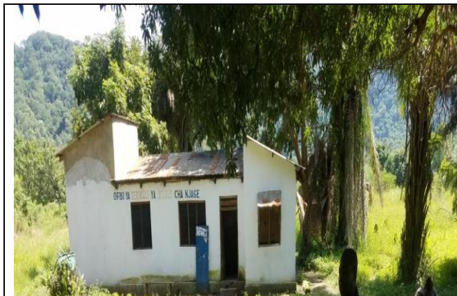
Photo2.17: Njage village office
